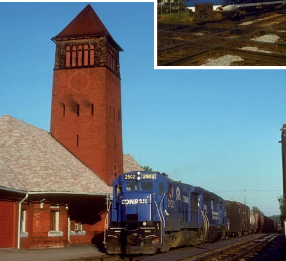
Right - Nichols tower in Battle Creek was built in 1905 to protect the crossing of the Michigan Central and Grand Trunk Western mainlines. It was equipped with a 24-lever frame that controlled switches, signals and derails and was named after the neighboring Nichols & Shepherd factory. The crossing would be eliminated in the 1980s when traffic on the former MC was re-routed over the Grand Trunk through downtown Battle Creek. On August 8, 1975 Amtrak turbo # 58 heads west past Nichols tower with train # 355.
