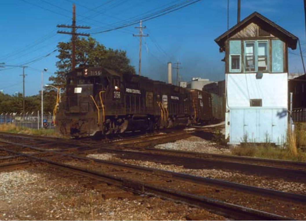
Right - Nichols tower in Battle Creek was built in 1905 to protect the crossing of the Michigan Central and Grand Trunk Western mainlines. It was equipped with a 24-lever frame that controlled switches, signals and derails and was named after the neighboring Nichols & Shepherd factory. The crossing would be eliminated in the 1980s when traffic on the former MC was re-routed over the Grand Trunk through downtown Battle Creek. On August 8, 1975 Amtrak turbo # 58 heads west past Nichols tower with train # 355.
