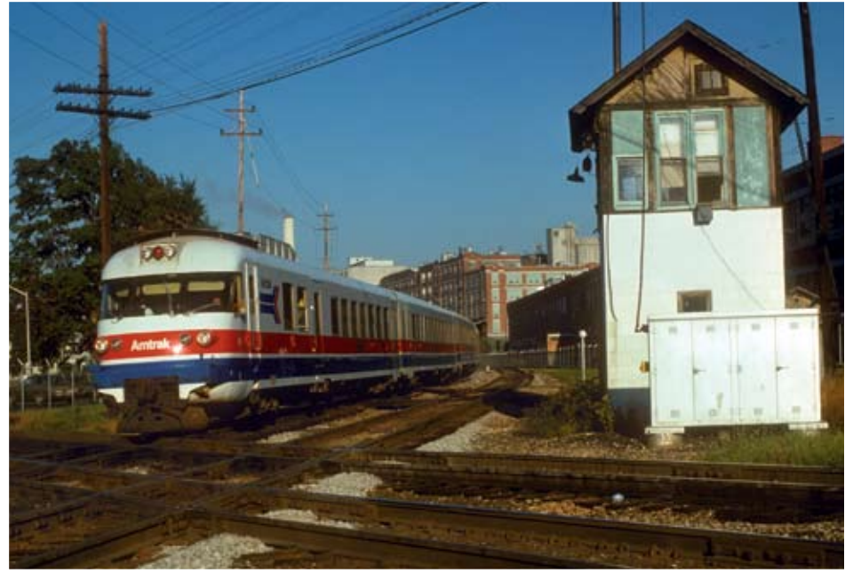
Right - Nichols tower in Battle Creek was built in 1905 to protect the crossing of the Michigan Central and Grand Trunk Western mainlines. It was equipped with a 24-lever frame that controlled switches, signals and derails and was named after the neighboring Nichols & Shepherd factory. The crossing would be eliminated in the 1980s when traffic on the former MC was re-routed over the Grand Trunk through downtown Battle Creek. On August 8, 1975 Amtrak turbo # 58 heads west past Nichols tower with train # 355.
